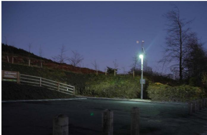
An LED Streetlight (together with a turbine, solar panel, occupancy and daylight sensor, battery and control system) is used in this application where there was no local electricity supply.
