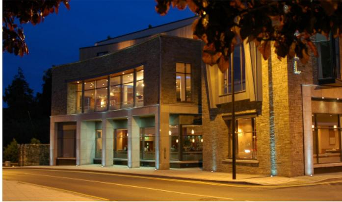
LED Groundlights used in this application are only 3w but have a narrow beam range of 5m to illuminate the pillars. They are also cold to touch (to prevent burning), have a 24v supply (safe if broken) and are a small size (less chance of breakage or trip hazard).
